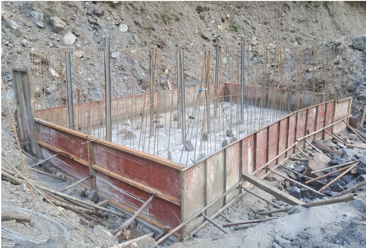
Figure 9: 1 st lift plum concreting in AB 9
