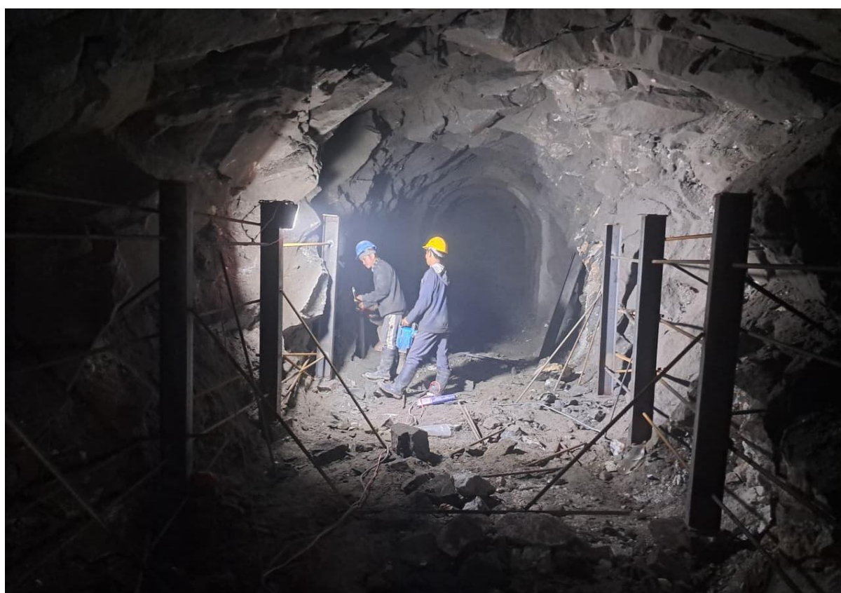
Figure 6: Rib installation work in Inlet tunnel
