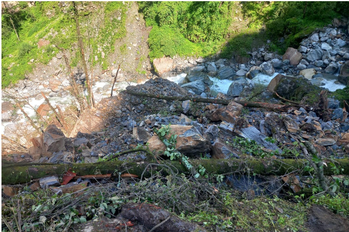
Figure 14: Powerhouse area after blasting
