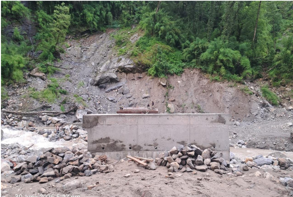
Figure 11: Bridge right abutment after removal of formwork
