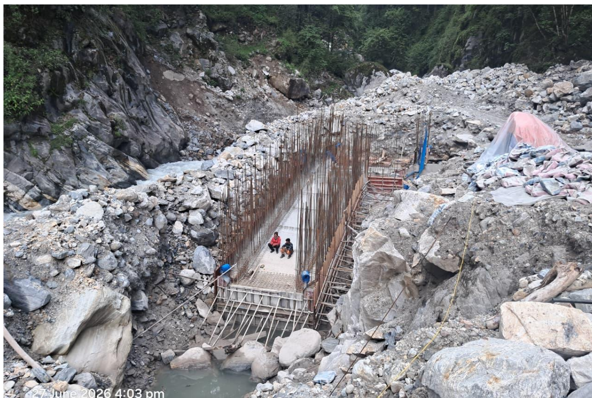
Figure 3: Undersluice gated panel after raft concreting
