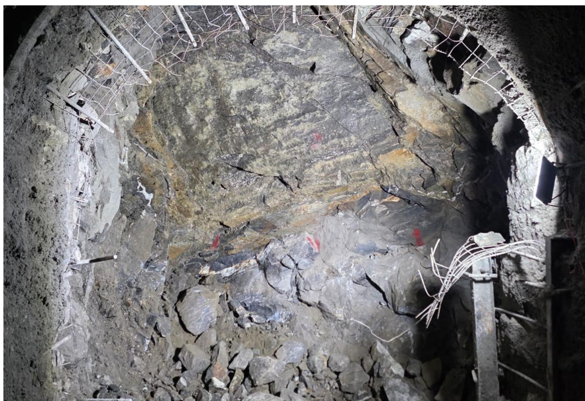
Figure 4: Inlet tunnel face at ch 0+053.60m
