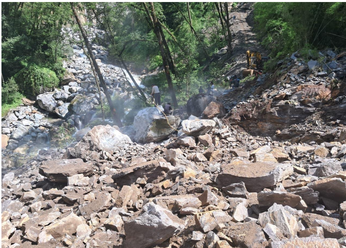
Figure 15: Drilling work for excavation in Powerhouse area
