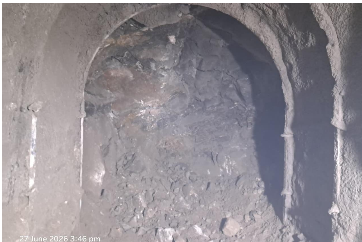
Figure 5: Face drilling in Inlet tunnel at ch 0+056.10m
