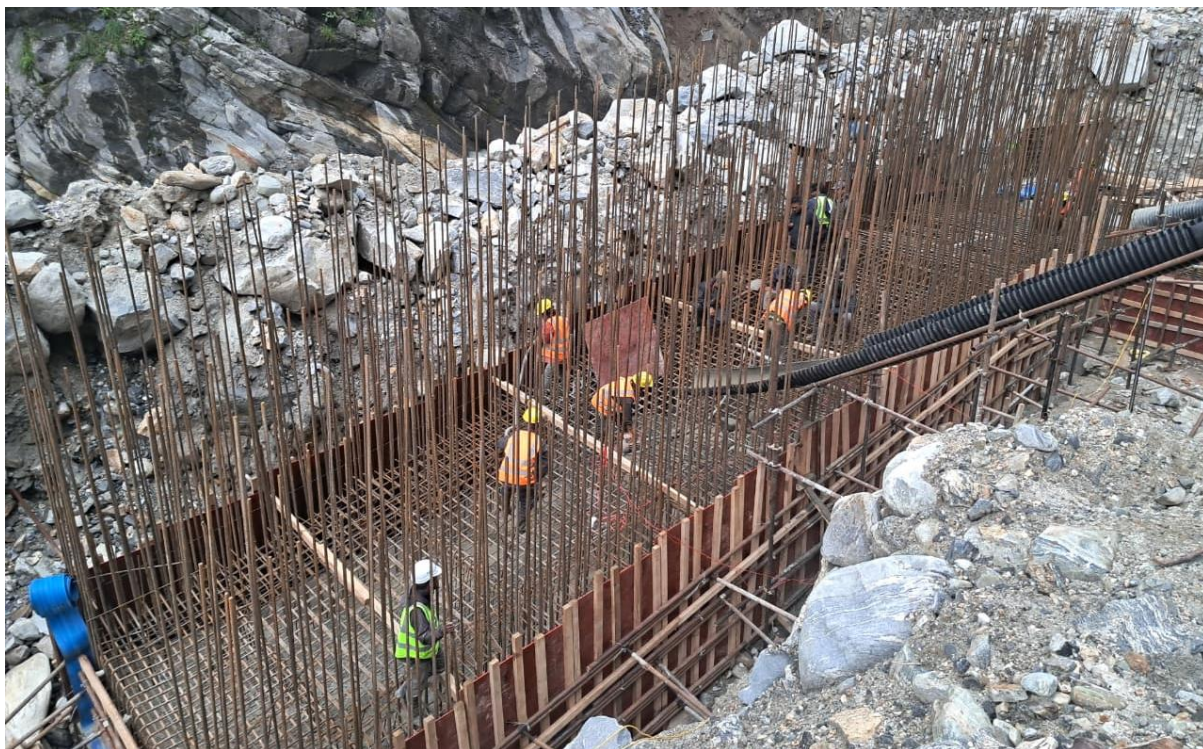
Figure 2: Rebar and formworks in Undersluice gated panel in Headworks
