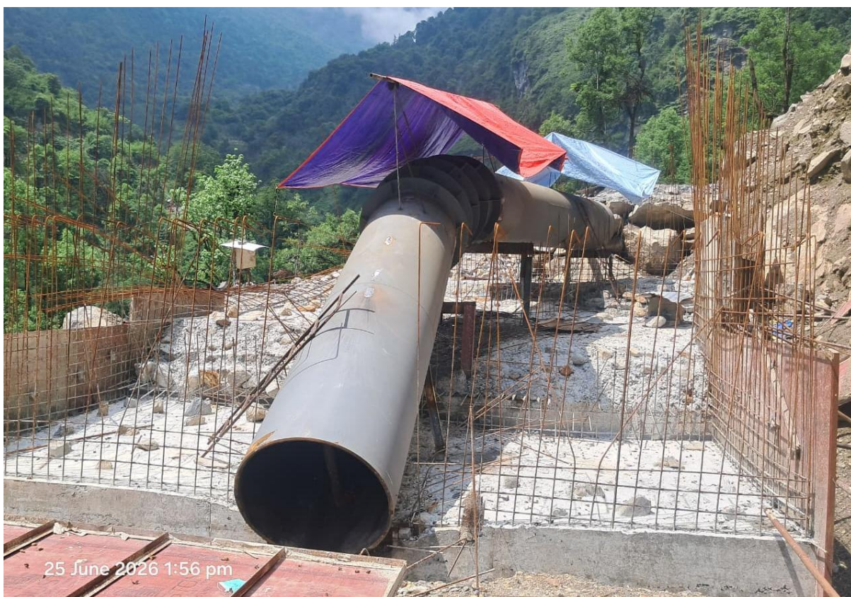
Figure 8: Bend and straight pipe erection completed in AB 12
