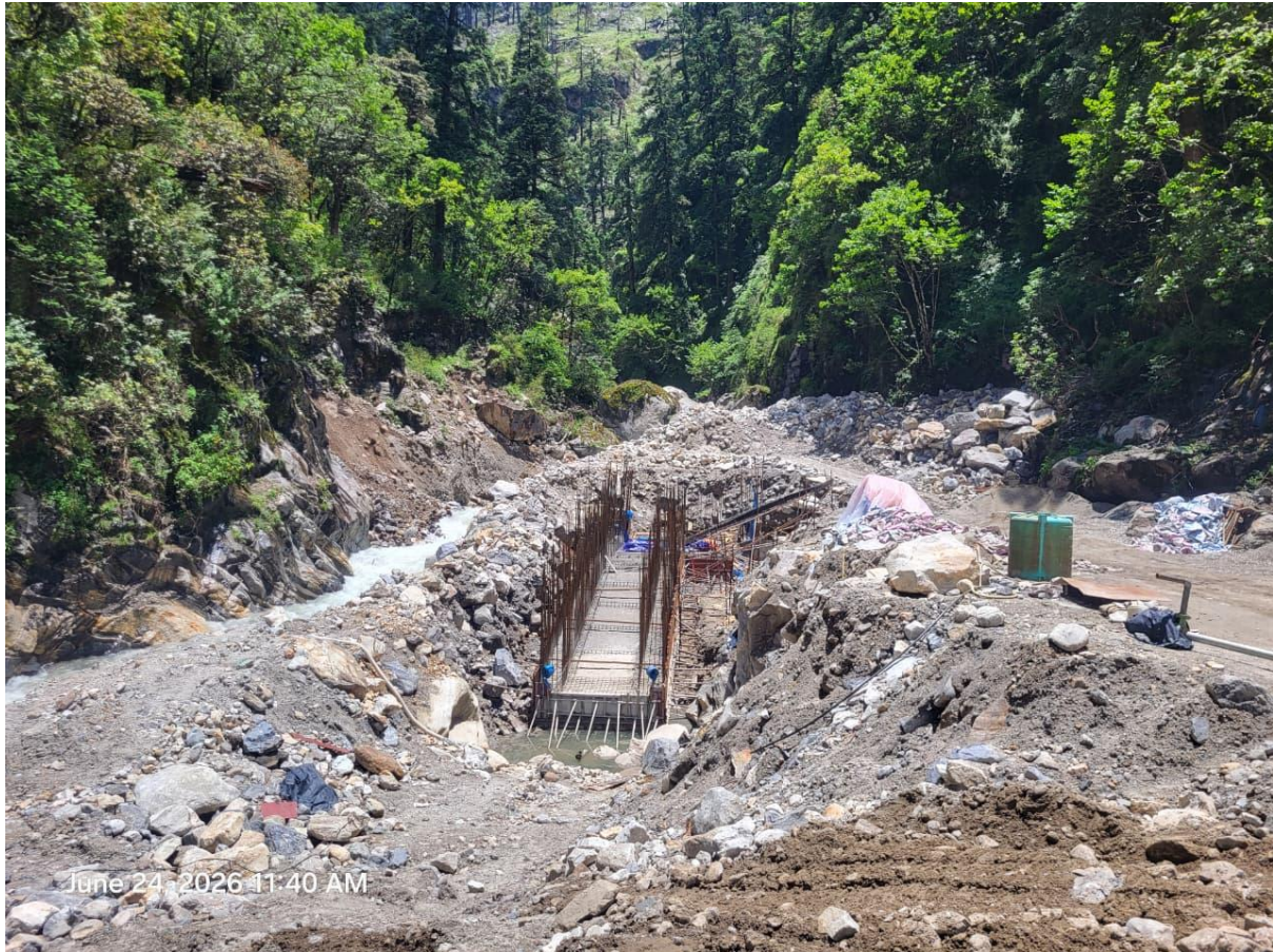
Construction of Nyadi Phidi Hydropower Project (21.4 MW)
