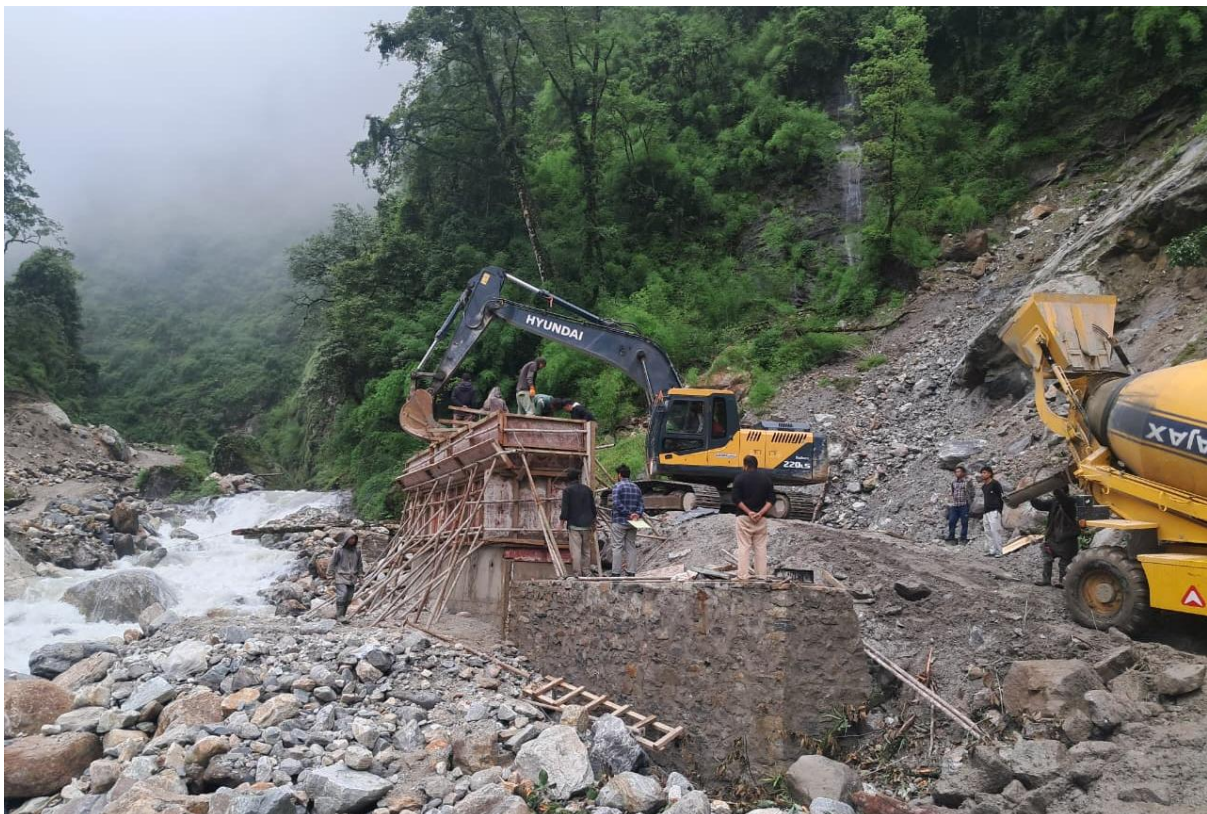
Figure 12: Concreting in Bridge left abutment stem wall
