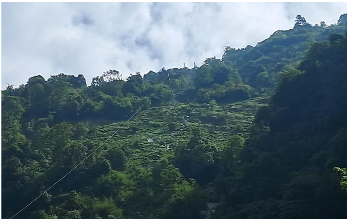
Figure 16: Rope tensioning of Ropeway
