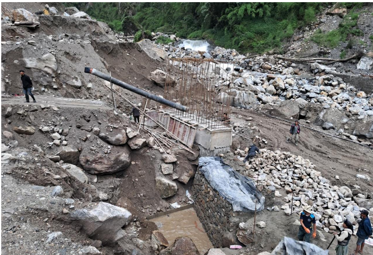
Figure 10: Stem wall along with RRM of bridge right abutment
